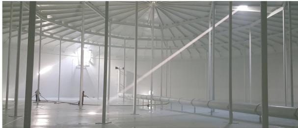
Recoating a potable water reservoir of this magnitude is a long and complicated process. All of the existing paint has to be sandblasted off and then the bare steel must be recoated, following careful processes to protect the environment. In addition, this reservoir needed a significant amount of welding work to prevent future corrosion on the roof of the structure.
