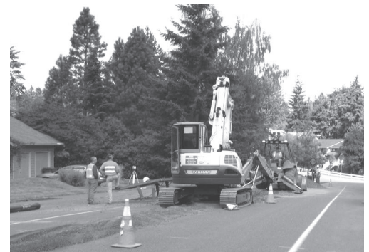
Sewer extension under construction
